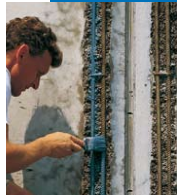
Application de Mapefer
